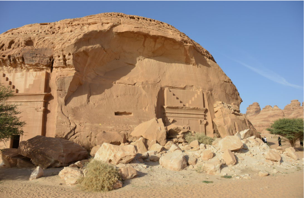
Hegra – Thermal stress, erosion and geomorphological instability in KSA © Spizzichino
